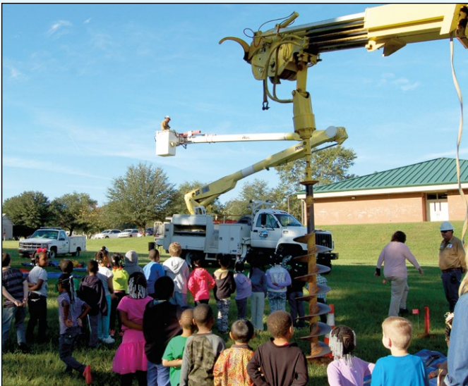
Eastside Elementary School students watch as LaFayette Electric Department apprentice Chris Sanders goes up in the city’s bucket truck.
