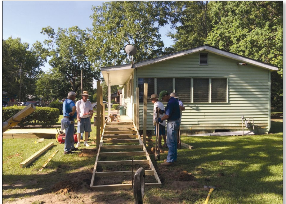
Ecumenical Ministry volunteers at work on a home repair project.
