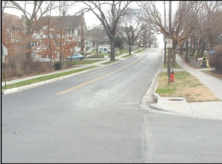
*Street transition (part 3)* – the same arterial street two hundred feet further up the street supporting residential land use. Expanded sidewalks and parking lanes have transitioned to expanded planting strips.
