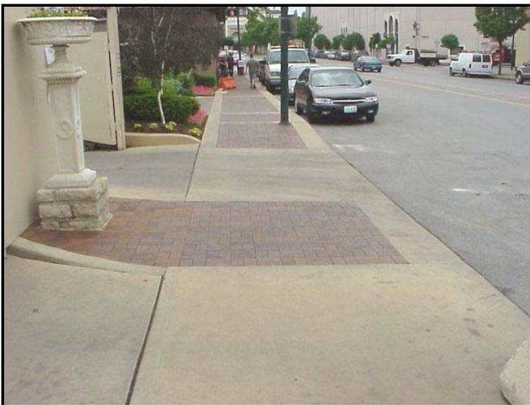
*Lot access* – Curb cuts that maintain a continuous sidewalk with a different material than the street and driveway on a commercial block.
