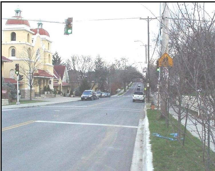
*Street Transition (part 2) – the same arterial street two hundred feet further up the street supporting an institutional land use. Angled parking has transitioned to parallel parking allowing a more narrow street and the addition of a planting strip and an expanded sidewalk in front of the church.*
