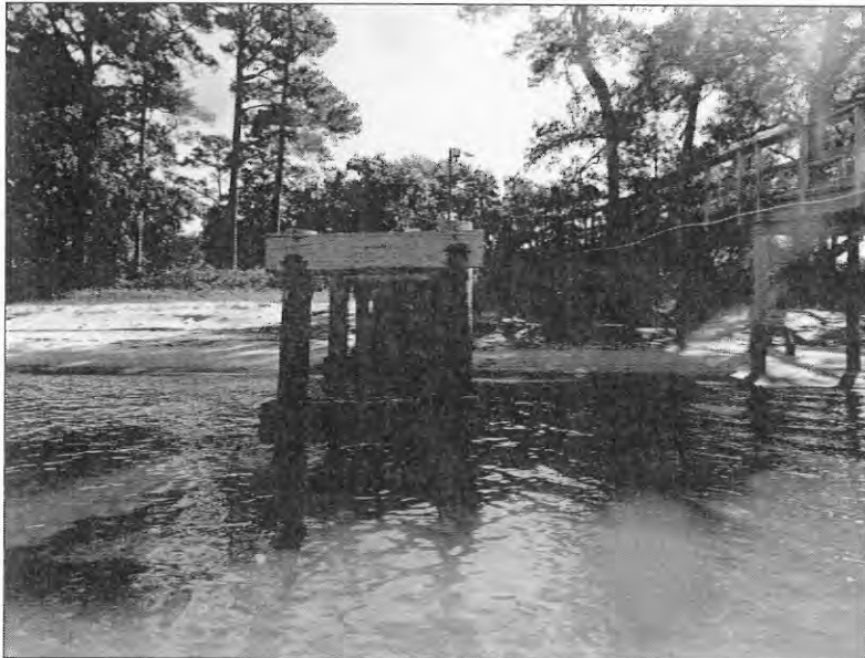
Pictured: Orange Street Pier storm drain pipe (Major Outfall # 8)
