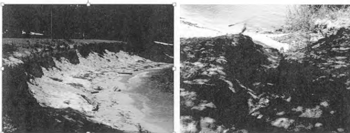
Pictured: Beach erosion at Magnolia Beach Park (Pier Street) after April 2014's storm events. ; Photo Credits: John Saraceno
