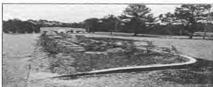
Pictured: Bio-detention at 451 Pecan Street (City building)
