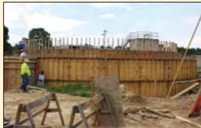
Construction of one additional aeration basin.
