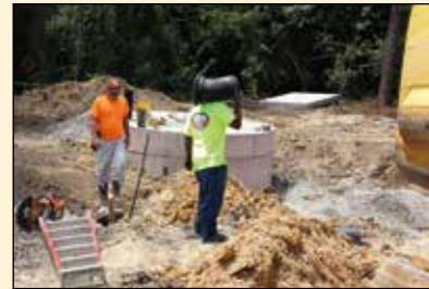
Crew members work on lift station number 2.
