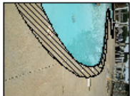
100' END OF POOL AREA OF CONCRETE REPAIR
