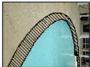
50' END OF POOL AREA OF CONCRETE REPAIR
