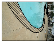
NORTH EDGE OF POOL AREA OF CONCRETE REMOVAL
