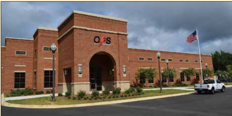
View of the Opelika Power Services office as you drive into the parking lot at 600 Fox Run Parkway.
