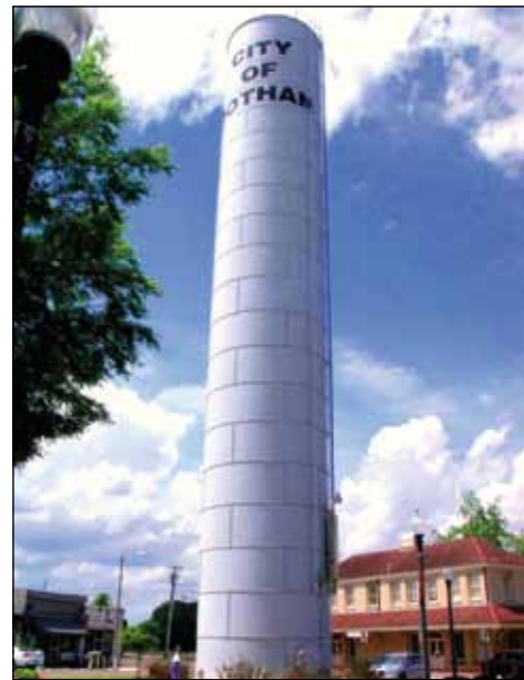
City of Dothan 'Dixie' Standpipe
