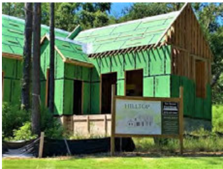
New Housing Construction in Fairhope (Hilltop)
