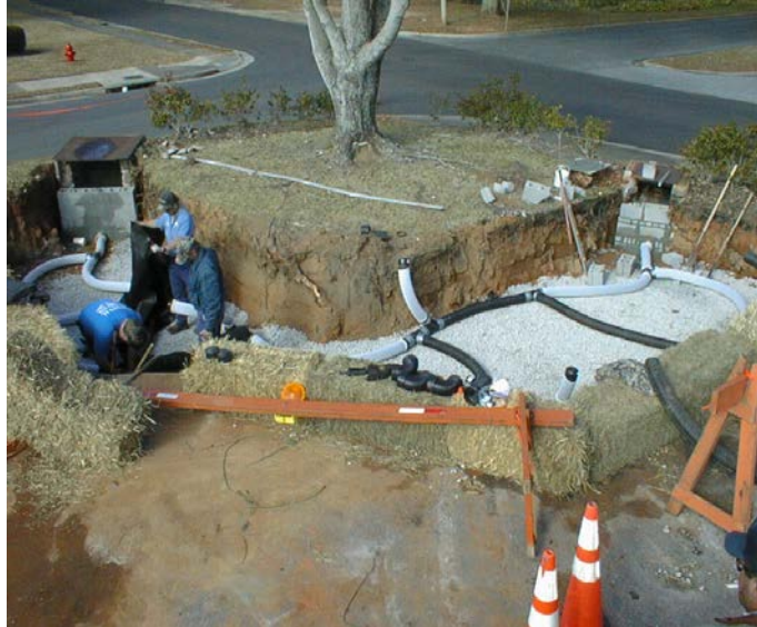
Pictured: Rain garden under construction at City Hall (2003)
