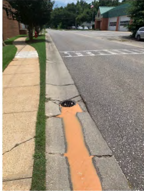
Figure 11: Turbid water running into storm drain
