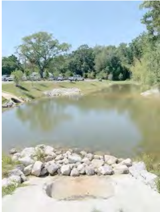
Figure 13: Outfall at The Reserve
