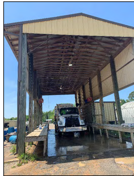
Figure 18: Public Works Wash Rack
