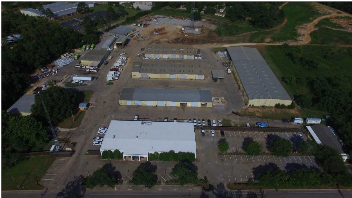
Aerial of Public Works Warehouse and Facility, 555 South Section Street
