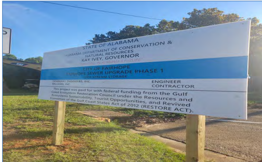
Pictured: Signage for sewer upgrade project, 2023/2024 (Tatumville Gully @ Public Works warehouse)
