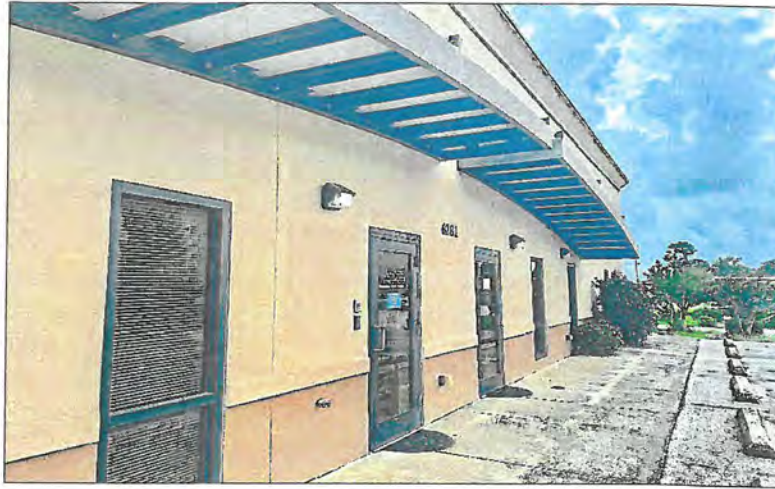
Automation Control Service – Primary Office
