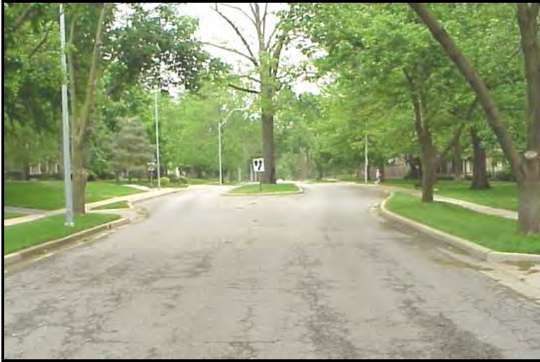
Traffic calming - Local street with center median.
