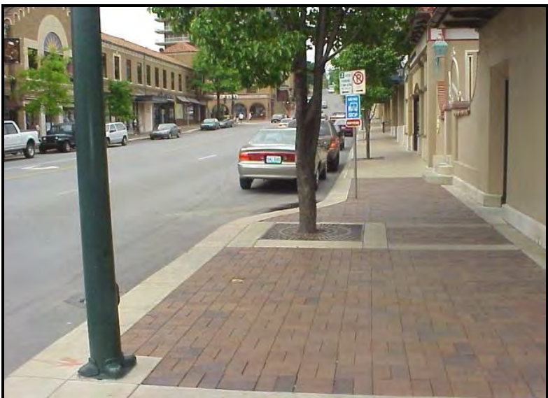
Traffic calming – Curb projection or bulb-outs creating space for on-street parking and narrowing the street at pedestrian crossing.
