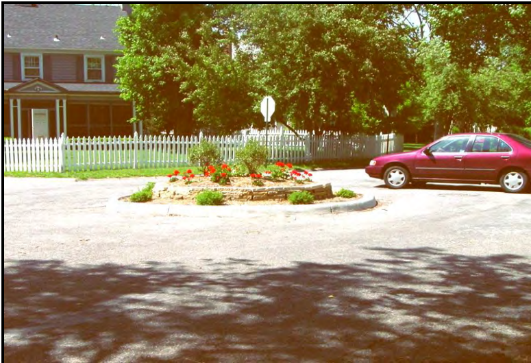
Traffic calming - Local street intersection with traffic circle.
