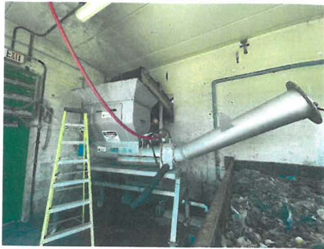
Figure 4-11: Typical Screenings Washing/Compacting Unit
