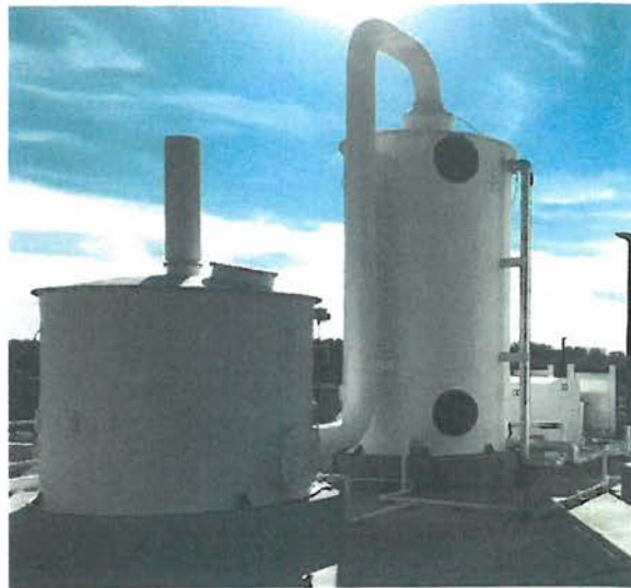
Figure 4-15: Typical Bioscrubber Odor Control System
