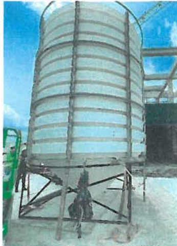
Figure 4-14: Modular Stacked Tray Vortex Grit Removal System
