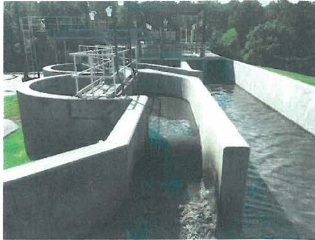
Figure 4-13: Typical Mechanically Induced Vortex Grit Removal System
