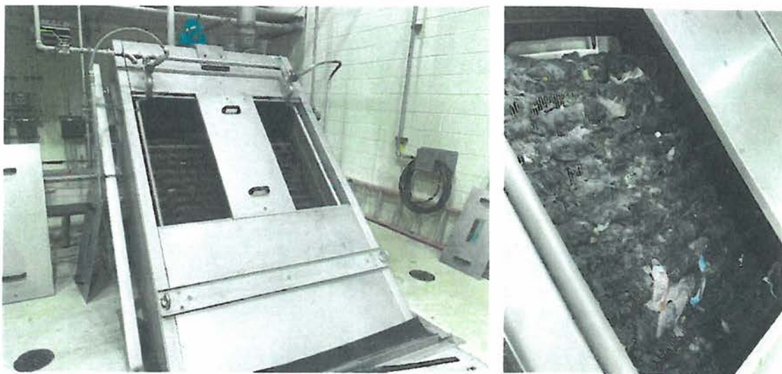
Figure 4-5: Typical Step Screen
