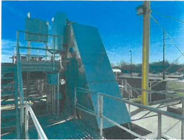
Figure 4-2: Typical Continuous Element Bar (Rake-Style) Screen
