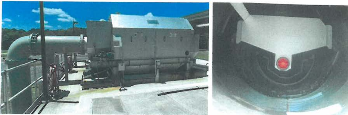
Figure 4-6: Typical Rotary Drum Screen
