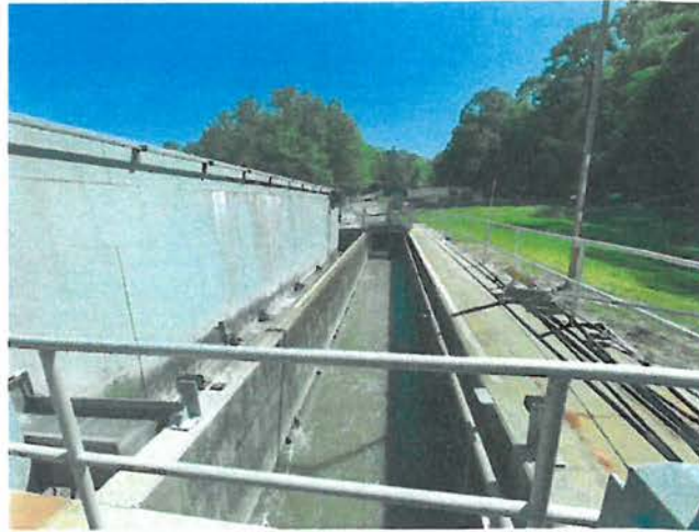
Figure 4-12: Existing Aerated Grit Removal System at the Fairhope WWTP
