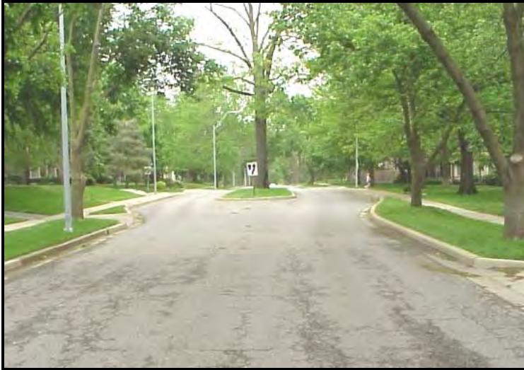
Traffic calming - Local street with center median.
