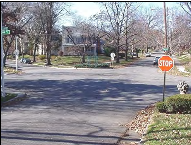
Intersections - Local street intersection with more than two local streets using 45 degree angle intersection.
