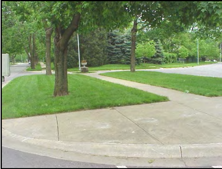
Intersections - Local street intersection with more than two local streets using median island and a series of 90 degree angle intersections.
