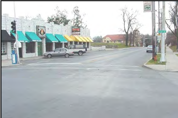
Street Transition (part 1) - Village center at the intersection of two arterial streets with angled and parallel on-street parking.
