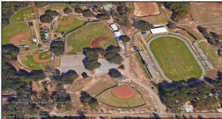
Figure 43 Volanta Gully outfalls are due for assessment in 2022, including the ones located in Volanta Sports Park
