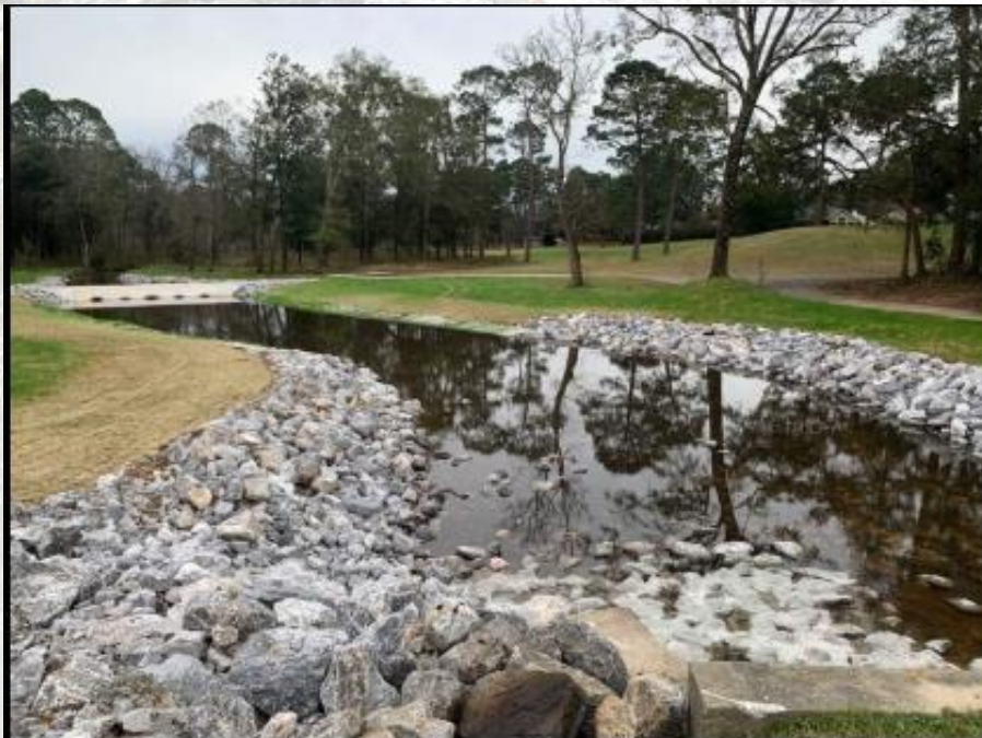
Figure 9 Quail Creek drainage improvement project, 2021
