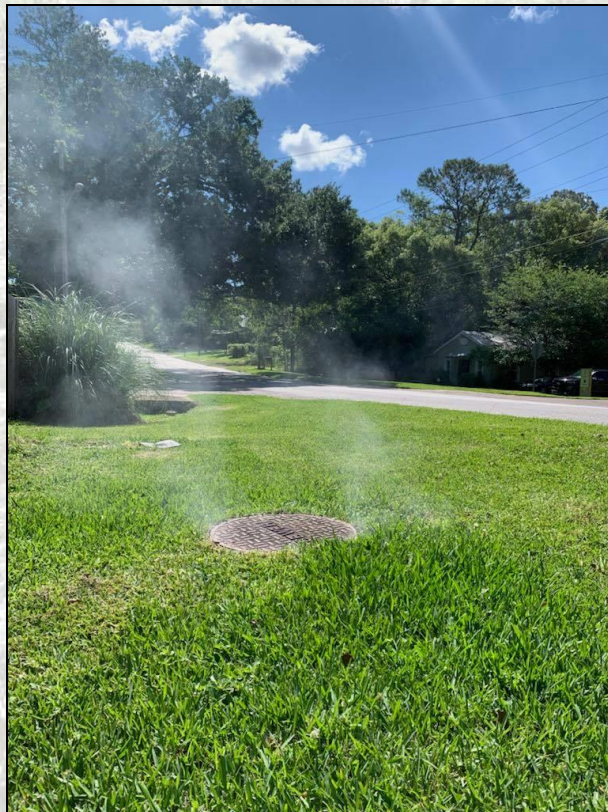
Figure 38 Example of smoke test
