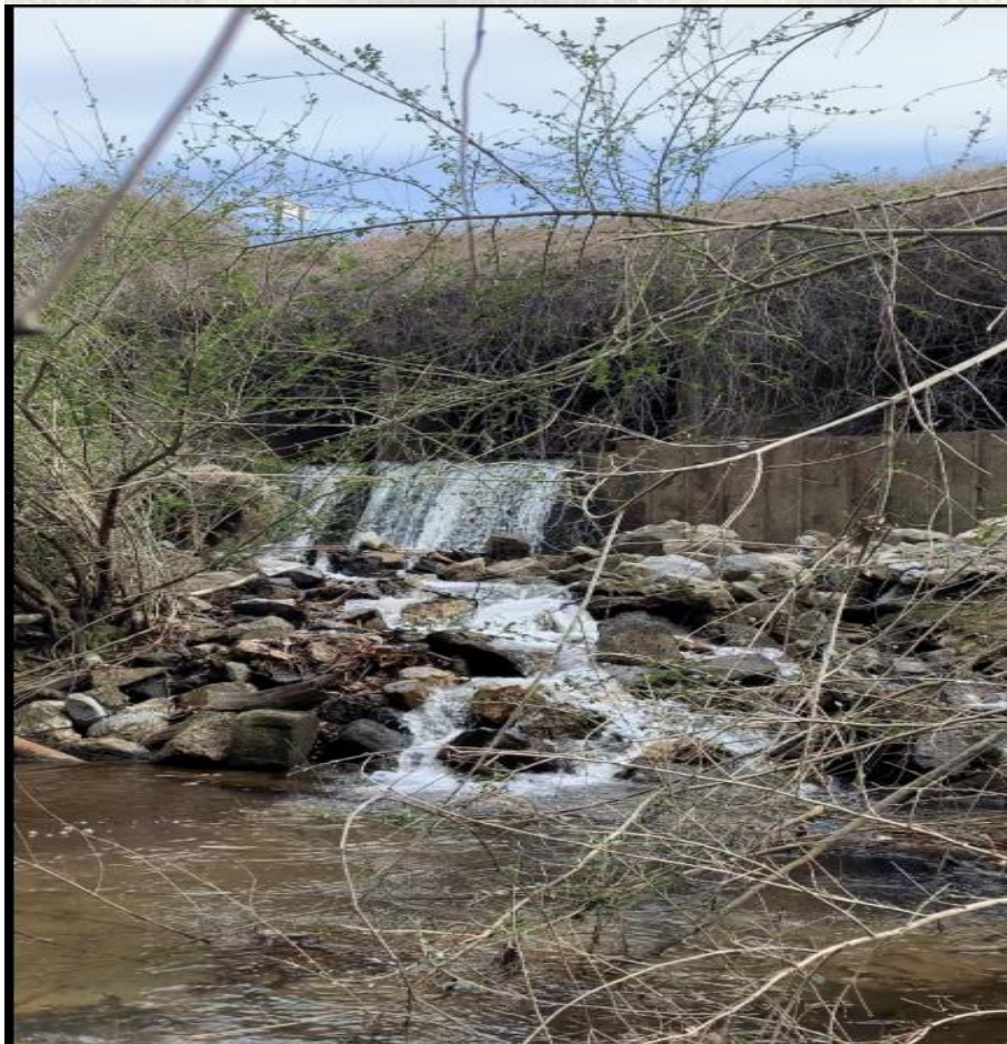
Figure 8 Fly Creek culverts at U. S. Highway 98
