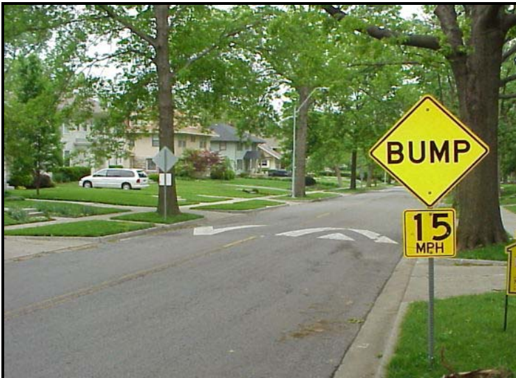
Traffic calming – Speed hump on collector street with residential uses fronting on street.
