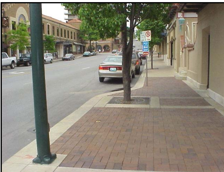
Traffic calming – Curb projection or bulb-outs creating space for on-street parking and narrowing the street at pedestrian crossing.
