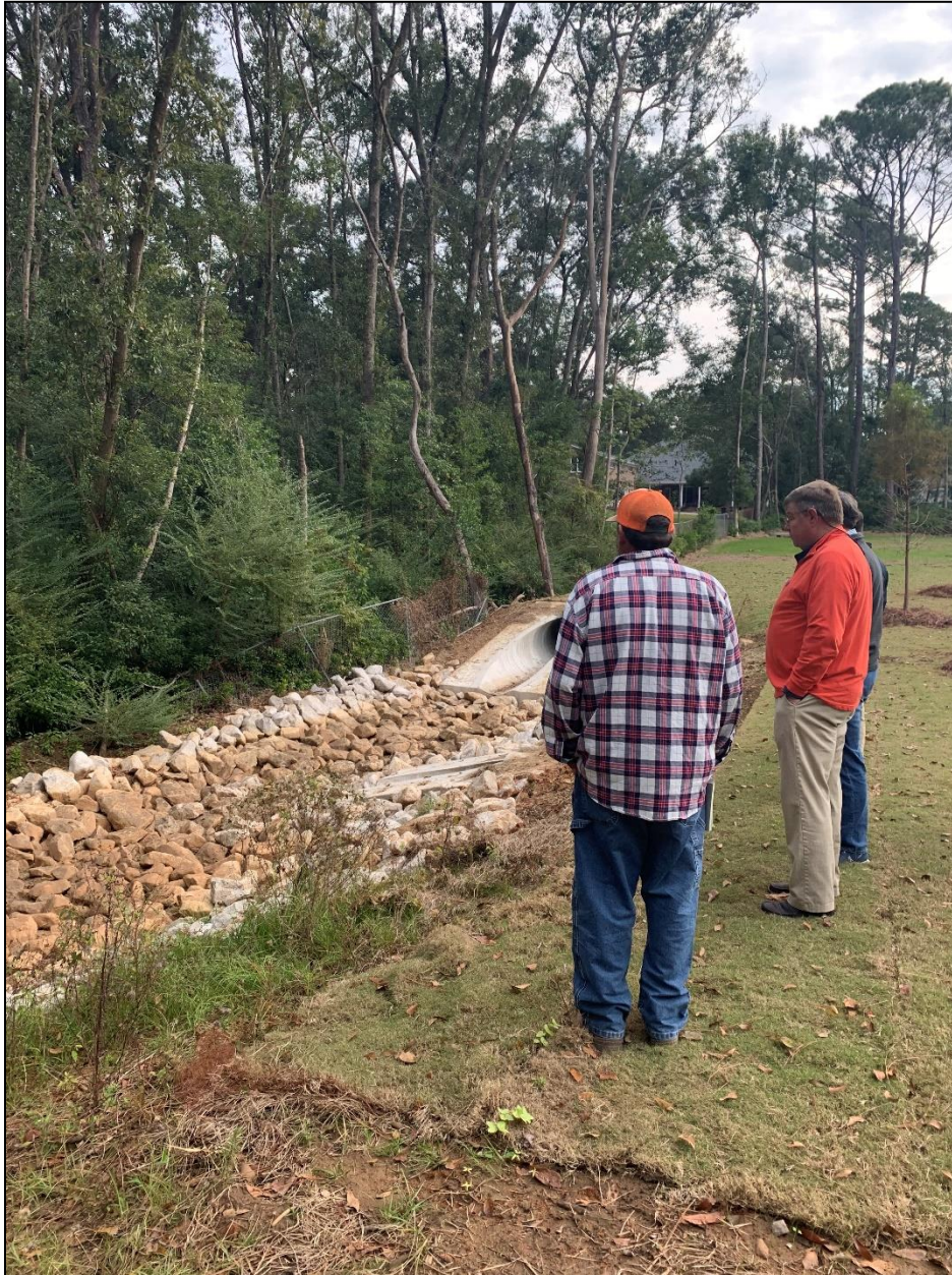
Figure 39 Stilling basins serve as a LID feature recently used in a development project “Hermitage Court”, Big Mouth Gulley watershed. Stilling basins also function as level spreaders per Public Works Director. November 2021
