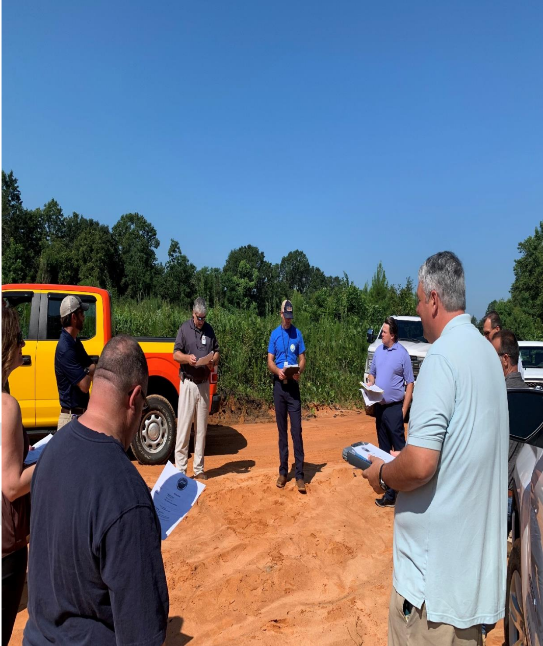
Figure 28 Pre-construction meeting on site with contractor and city staff to review construction procedures, including erosion and sediment control (Fox Hollow Phase 3, 2021)
