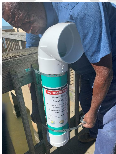
Figure 9: Public Works staff installed monofilament line recycling bins on the Fairhope Pier. Fairhope High School environmental clubs oversee collecting materials weekly.
