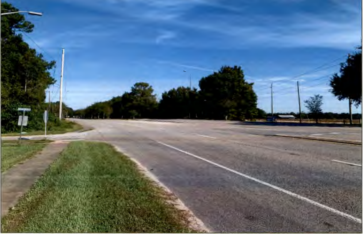
VIEW TO THE SOUTH – On US Hwy 98 looking towards the intersection with Volanta Ave
