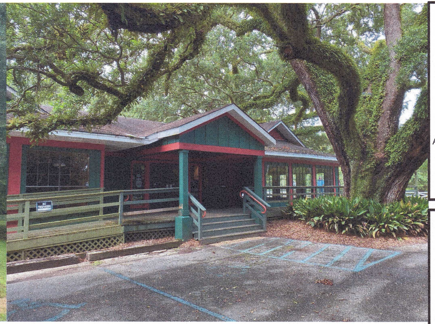
Existing Entrance and ADA Parking
