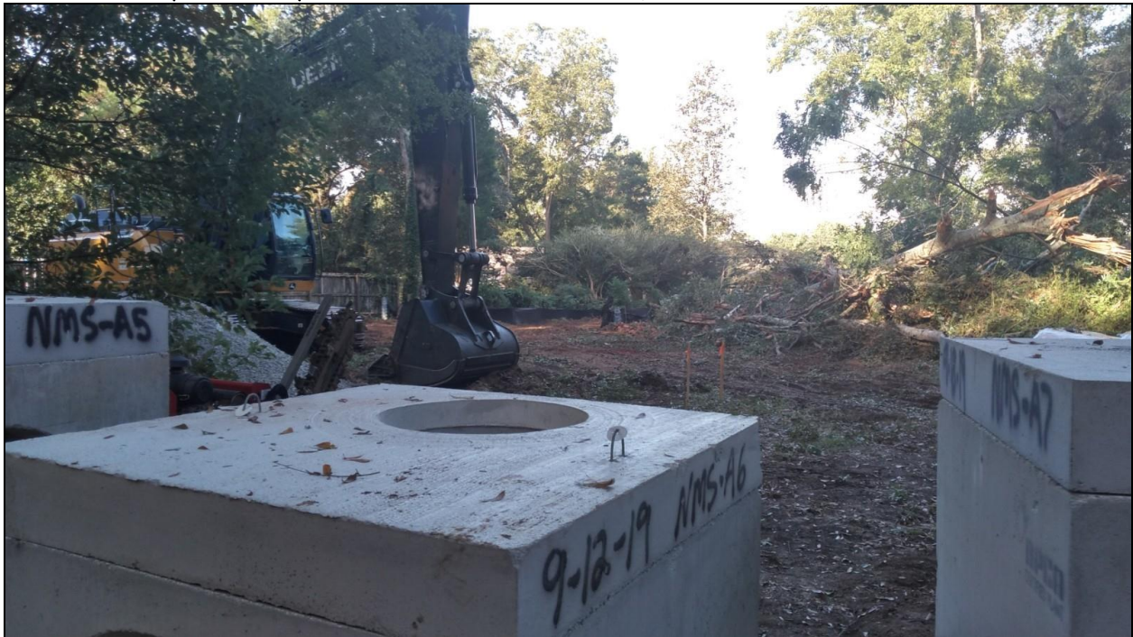
Figure 49 City stormwater project on North Mobile Street
