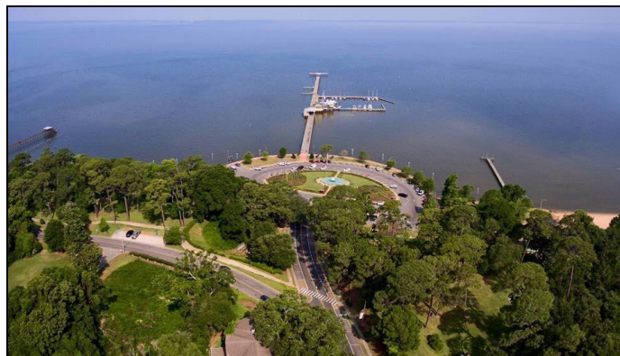
Figure 1 Fairhope Municipal Pier
