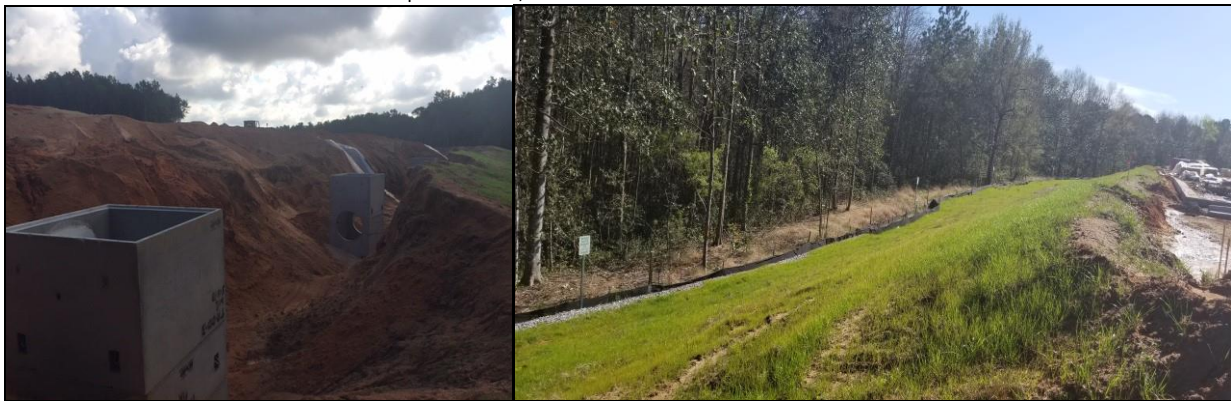
Figure 46 Level spreader installation (LID feature) at apartment complex project
