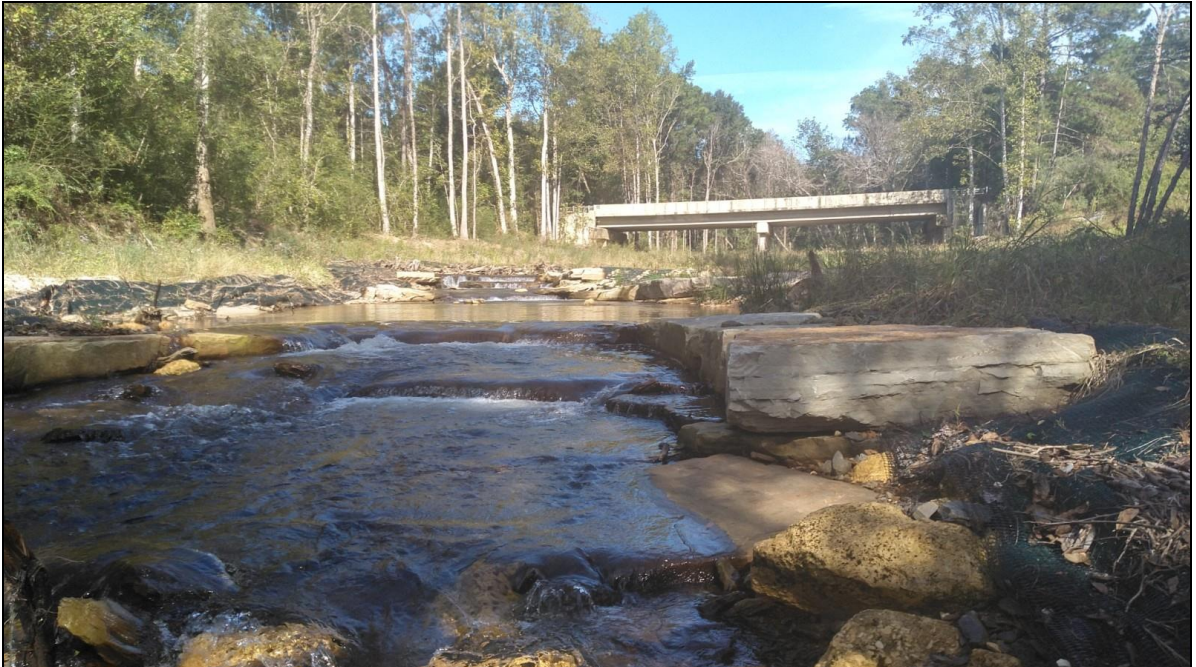
Figure 6 Rock Creek streambank stabilization project, Rock Creek Parkway, November 2019
