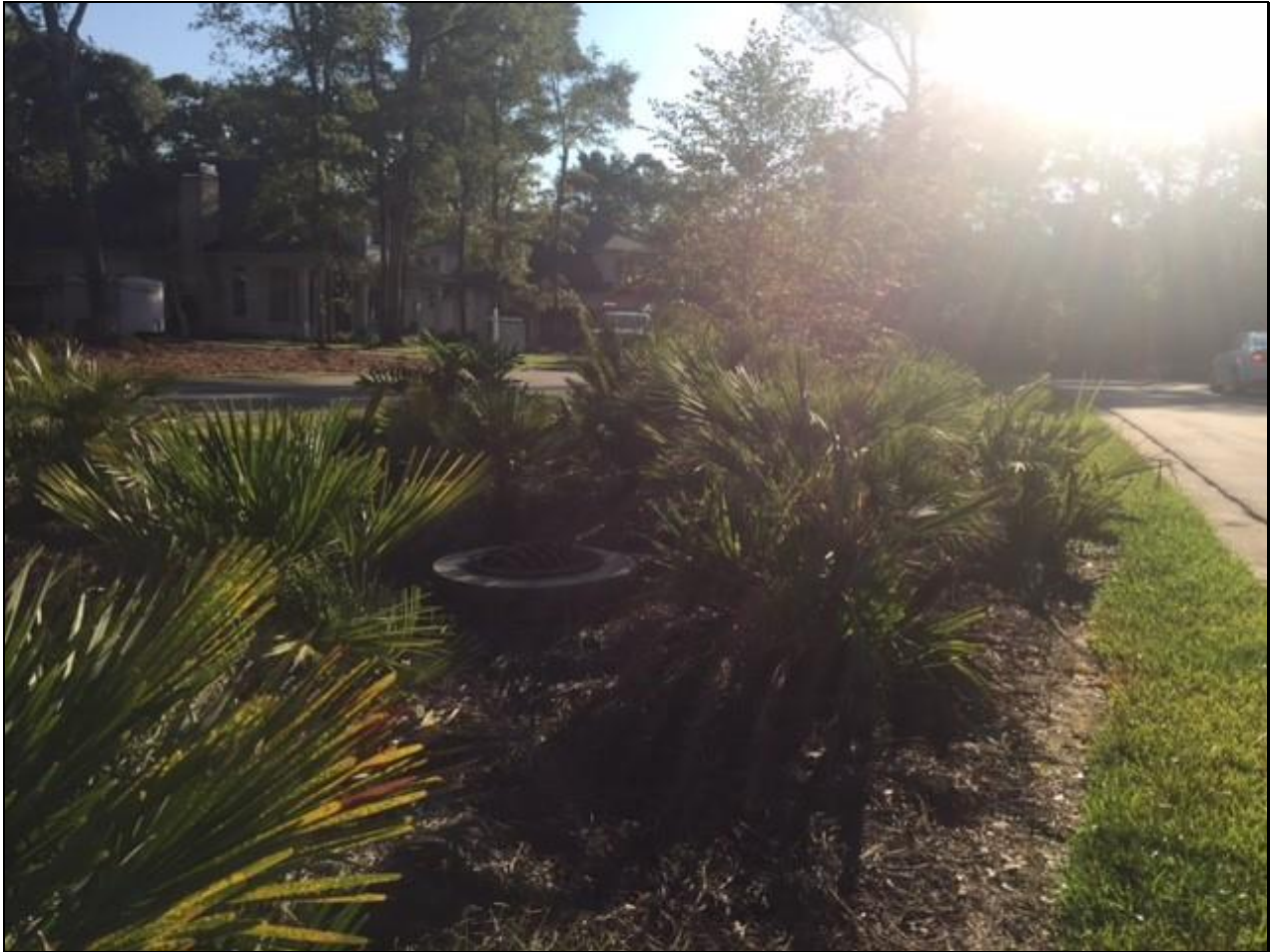
Figure 48 Example of a LID bio-swale stormwater facility in Fairhope subdivision
