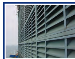
Enduro FRP/GRP louvers on an offshore platform off the Gulf Coast
