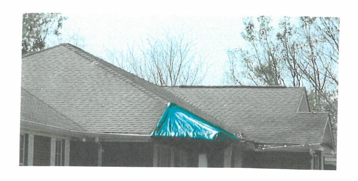
Localized roof damage- may repair just area impacted
