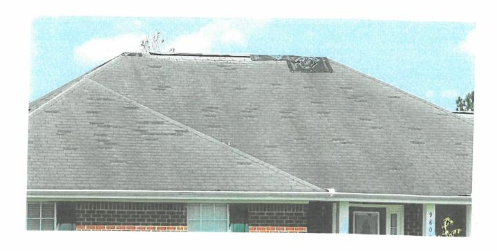
Distributed damage, will require complete re-roof and installation of sealed roof deck
