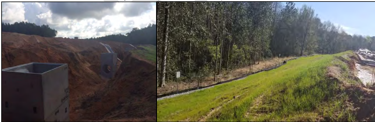
Figure 35 Level spreader installation (LID feature) at apartment complex project
