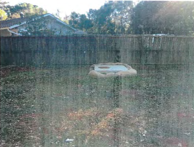
Looking south along border between lot 1 and 2 with drainage structure within the drainage and utilities easement.
