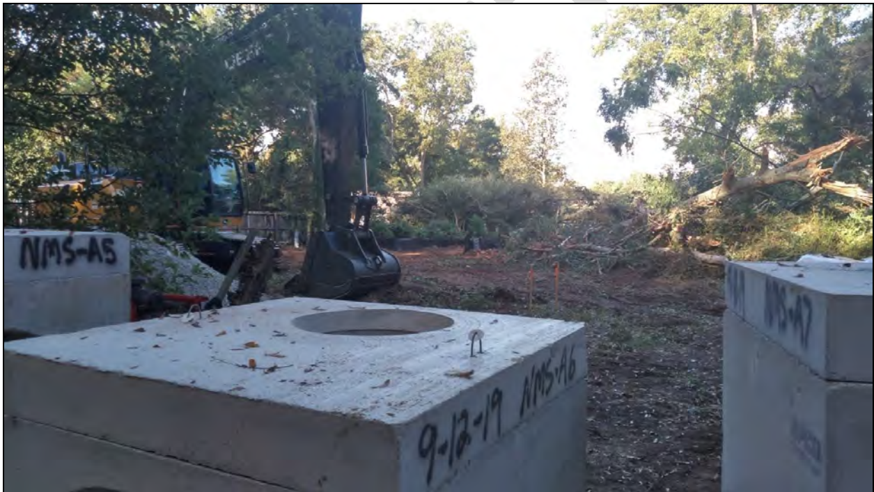
Figure 38 City stormwater project on North Mobile Street
