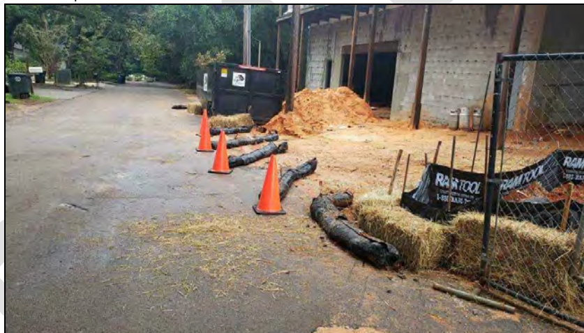
Figure 28 BMP Inspection: Notice of violation issued for BMP deficiencies (10/19)
