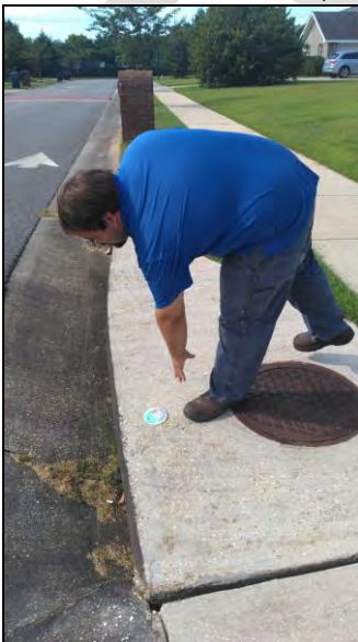
Figure 10 Public Works employee installing storm drain medallion
