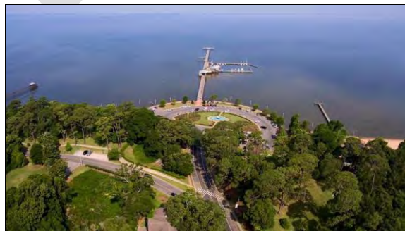
Figure 1 Fairhope Municipal Pier
