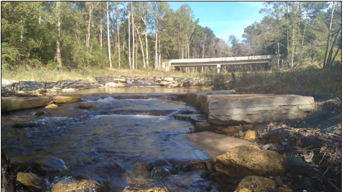
Figure 4 Rock Creek streambank stabilization project, Rock Creek Parkway, November 2019
