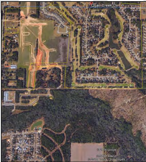
Figure 34 A sample subdivision undergoing site work in Fairhope's largest watershed, Cowpen Creek
