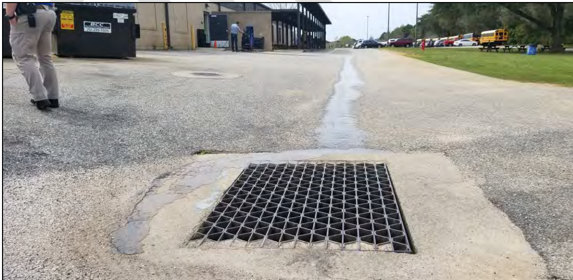
Figure 18 Example of illicit discharge: greasy water entering drain after cafeteria garbage can was rinsed in area discharging to storm drains, untreated
