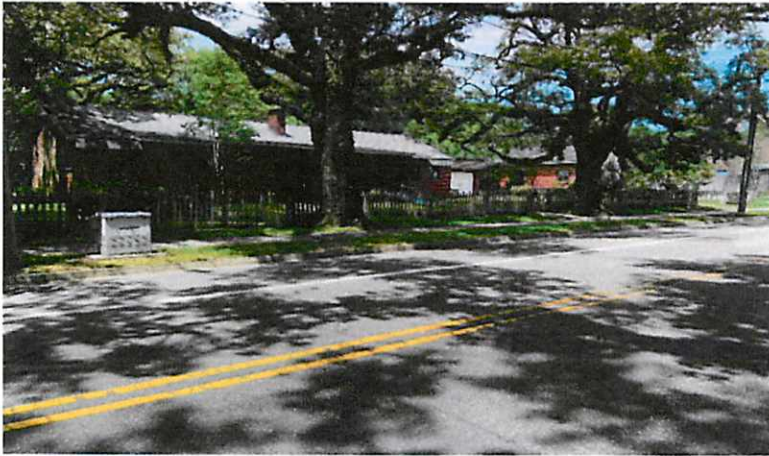
Subject Property looking northeast from across street on Fels Ave.
