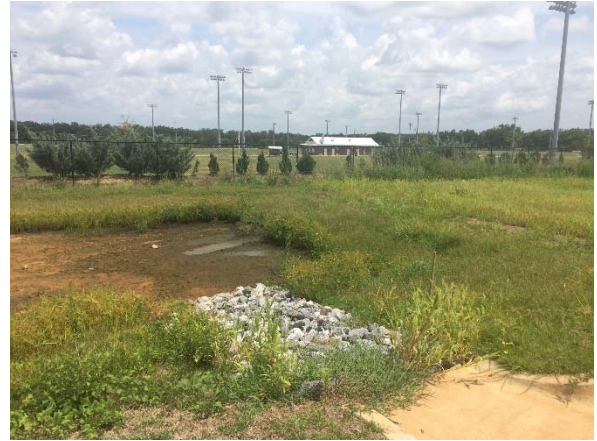
Looking southeast toward soccer complex from eastern terminus of Dutch Road
