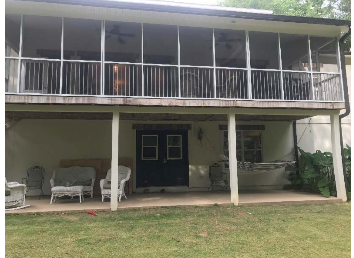
View of patio/covered porch
