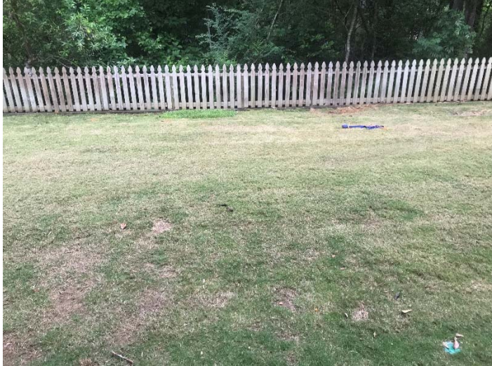
View of retaining wall and usable back yard.
