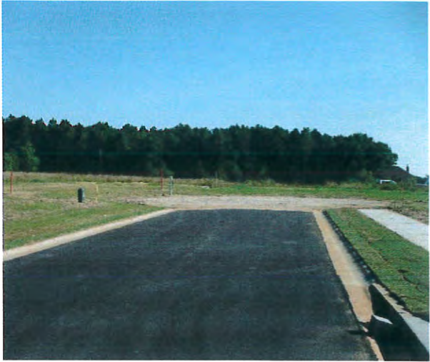
View toward the north side of site
