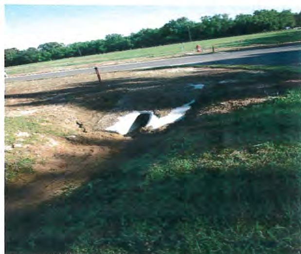
View looking south of swale along Lawrence Rd.
