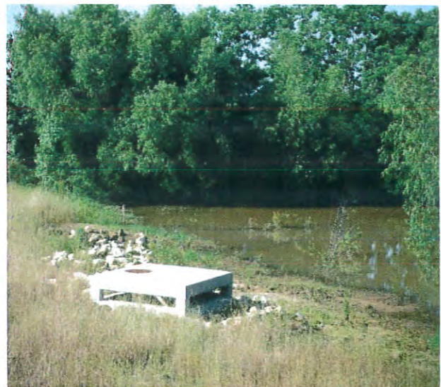
View of area of rip rap
