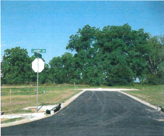
View to west (temporary turn around).
