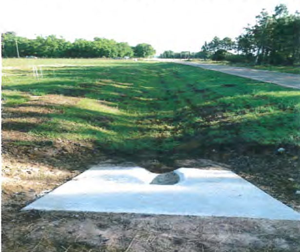
View looking north of swale along Lawrence Rd.
