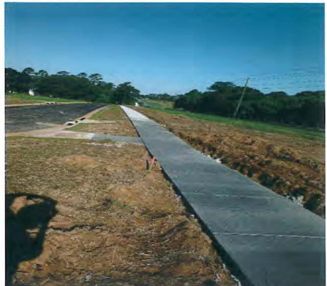
Sidewalk in common area along Hwy. 104.
