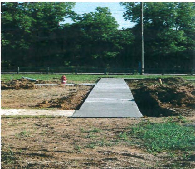
View of poured sidewalk.
