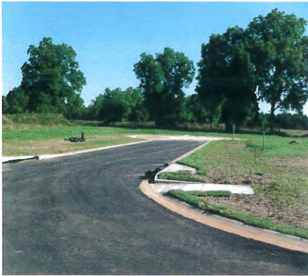
View of traffic circle (Sophie Falls Ave.)
