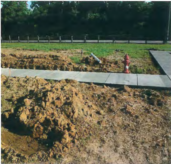
Sidewalk poured after final inspection.
