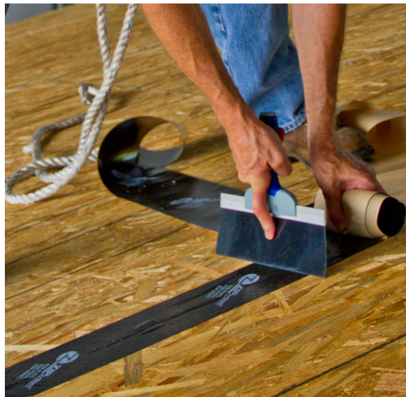
Figure 0-2. Applying qualified tape to roof deck seams using flat blade to eliminate voids and wrinkles.
