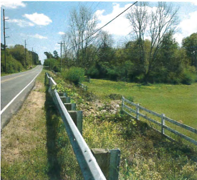
View of drainage rip rap across from site.
