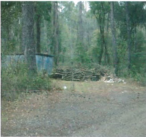
Staging area Battles Trace Phase 6
