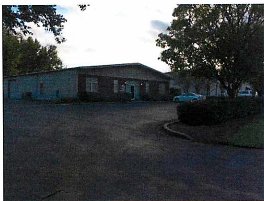
Subject property looking southwest from Nichols Ave
