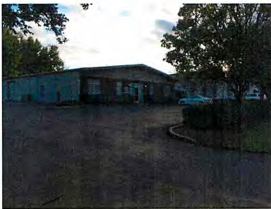
Subject property looking southwest from Nichols Ave
