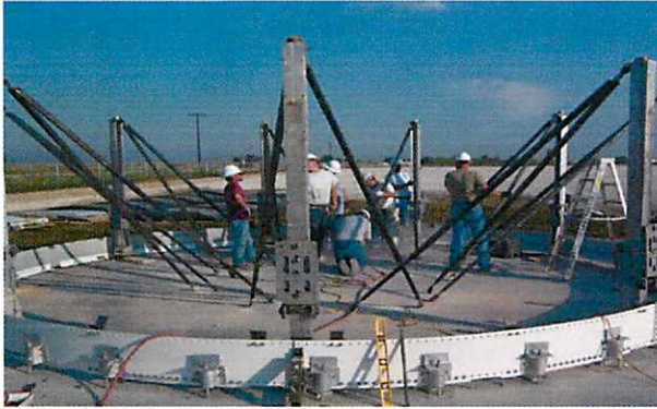
Dry Bulk Tank – Base Anchor Ring
