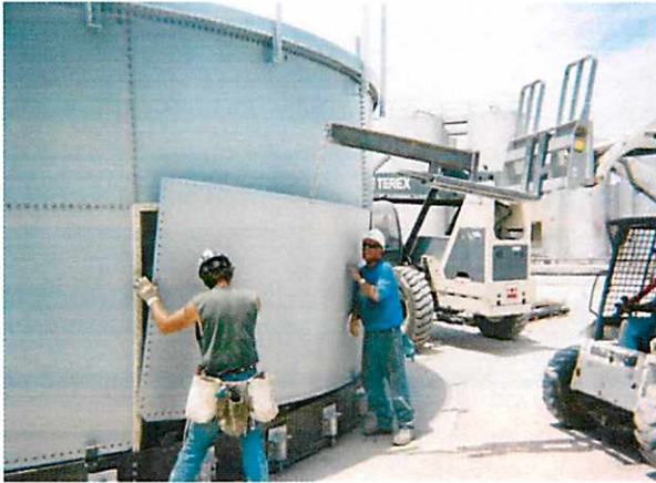
Dry Bulk Panel Installation
