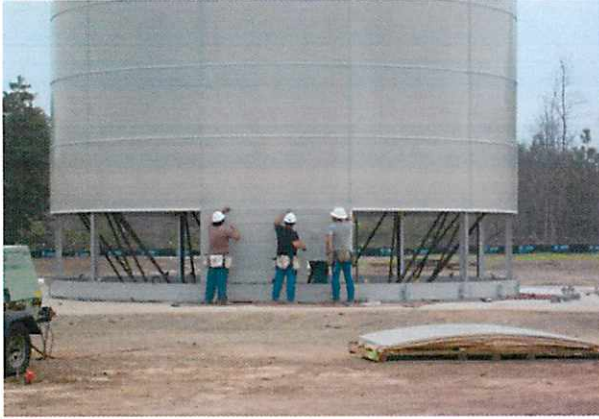
Dry Bulk Hopper Tank
