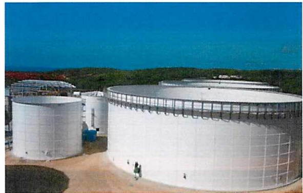
Anaerobic Digester Tanks
