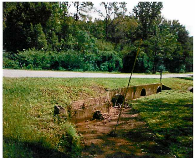
Backside of Culvert, with view of subject parcel.
