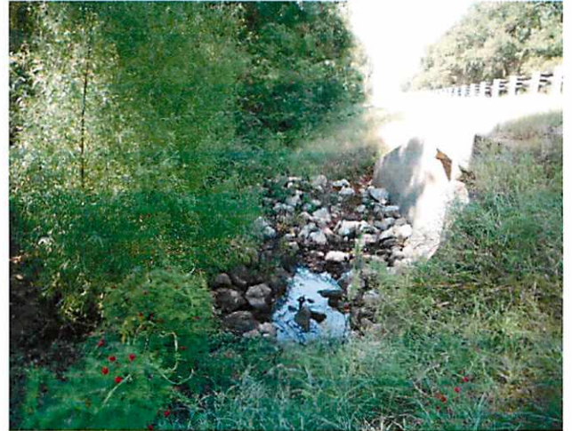
View of Culvert on property on Hwy. 104
