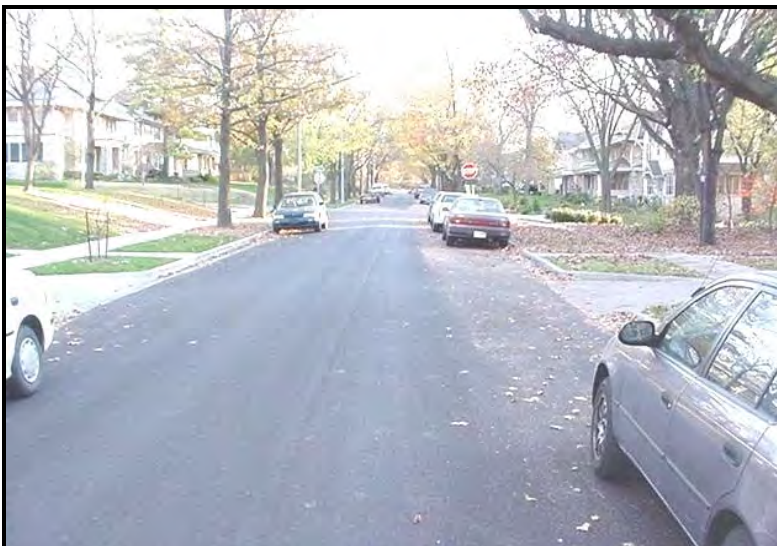
Street design - Local street with 1 yield flow lane and on-street parking on each side.
