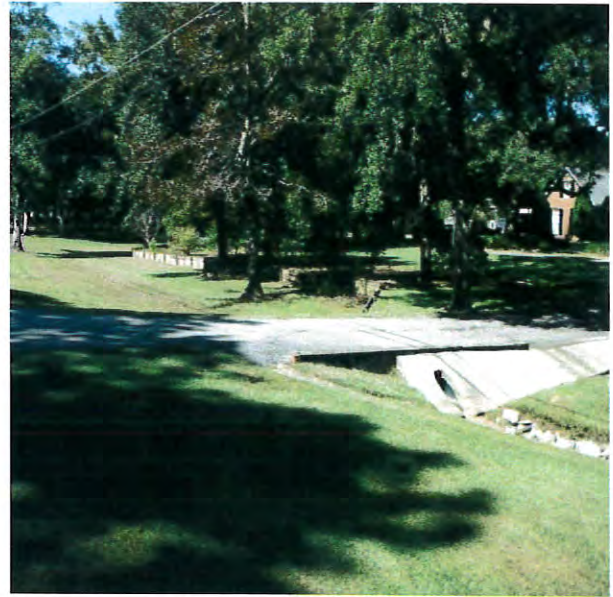
Culvert and drainage way shown on property.
