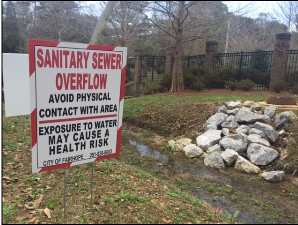
Pictured: Tatumville Gully notification of SSO (Middle Street @ Valley Street)
