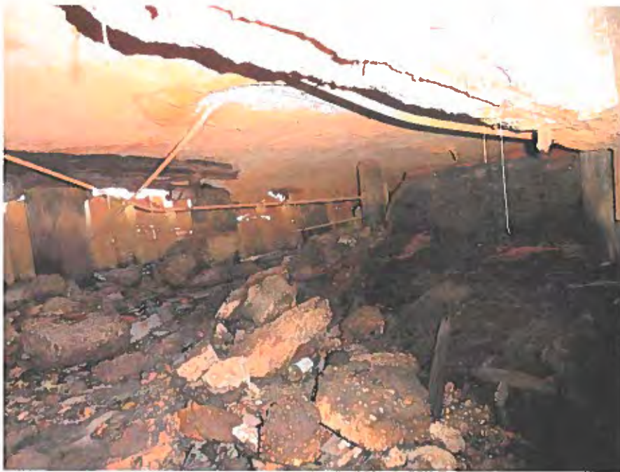
PHOTO 9 –SLAB UNDERMINING – EAST SIDE (FINGER PIER No. 2)
