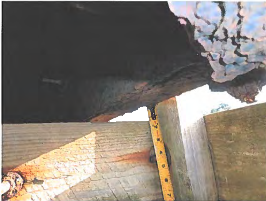
PHOTO 4 -BOTTOM BEAM FLANGE- LACK OF BEARING- INSIDE FLANGE (TYP)
