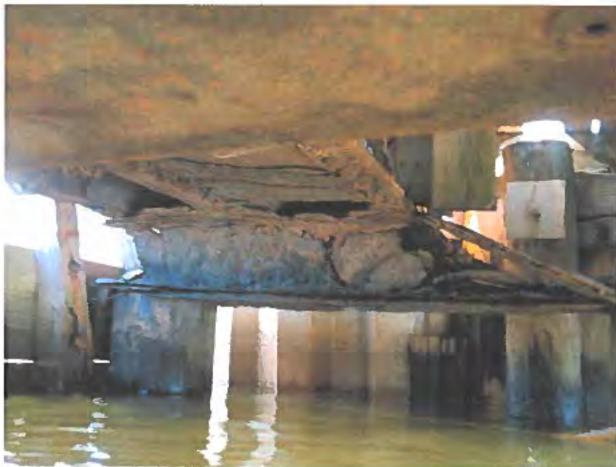
PHOTO 8 –STEEL CAP AT BENT NO. 8 – CRITICAL SECTION LOSS
