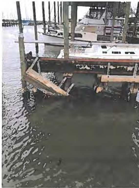
PHOTO 14 - FAILED FENDER SYSTEM – FINGER PIER 1 (TYP)
