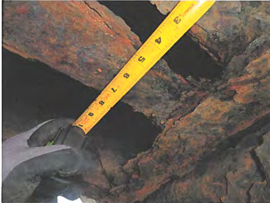
PHOTO 3 -BOTTOM BEAM FLANGE- SECTION LOSS UP TO 1" (WIDTH)
