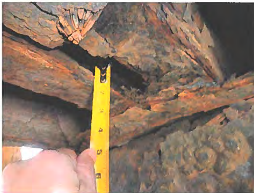
PHOTO 2 -BOTTOM BEAM FLANGE- SECTION LOSS UP TO ¼" TO KNIFE EDGE (TYP)
