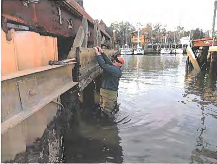
PHOTO 13- FAILED FENDER SYSTEM (TYP)
