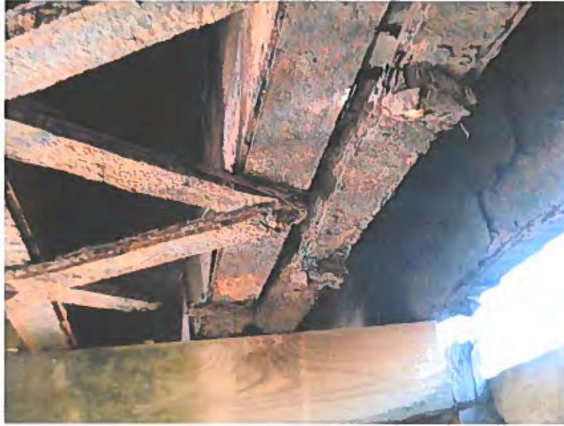
PHOTO 5 -BOTTOM BEAM CROSS BRACING (TYP)
