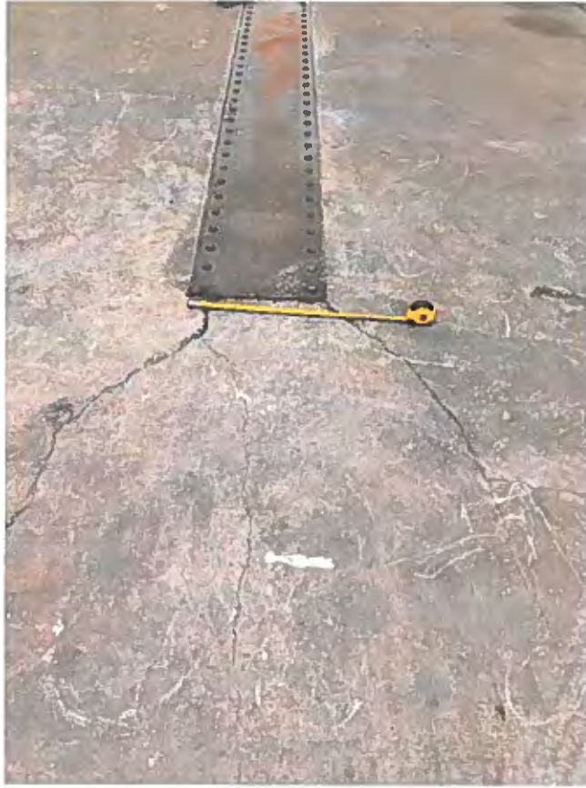
PHOTO 11 –TERMINUS OF BEAM B – CLASS 5 CRACKS (TYP)
