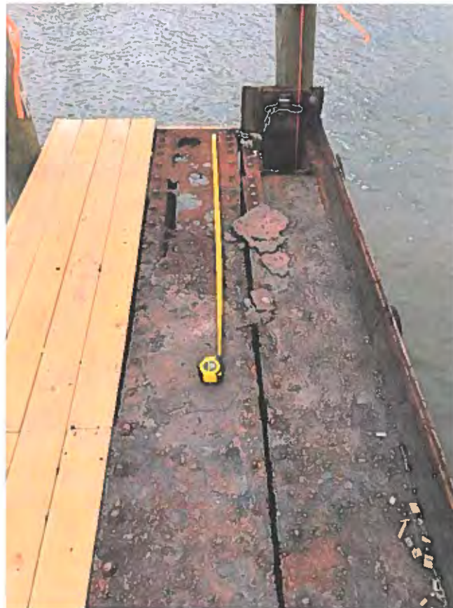
PHOTO 6 - FINGER PIER NO. 2 –BEAMS C AND D CRITICAL SECTION LOSS IN TOP PLATE
