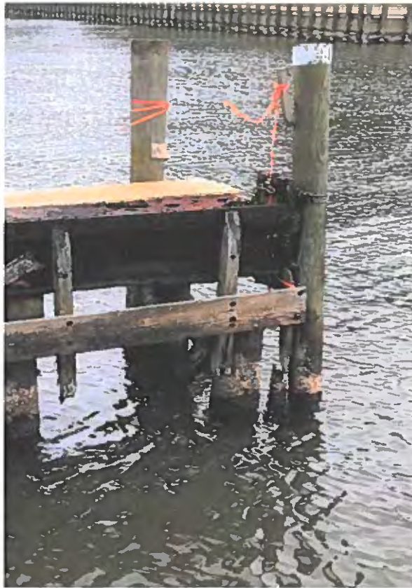
PHOTO 7 –FINGER PIER NO. 2 ; BENT CAP NO. 2 - MISSING
