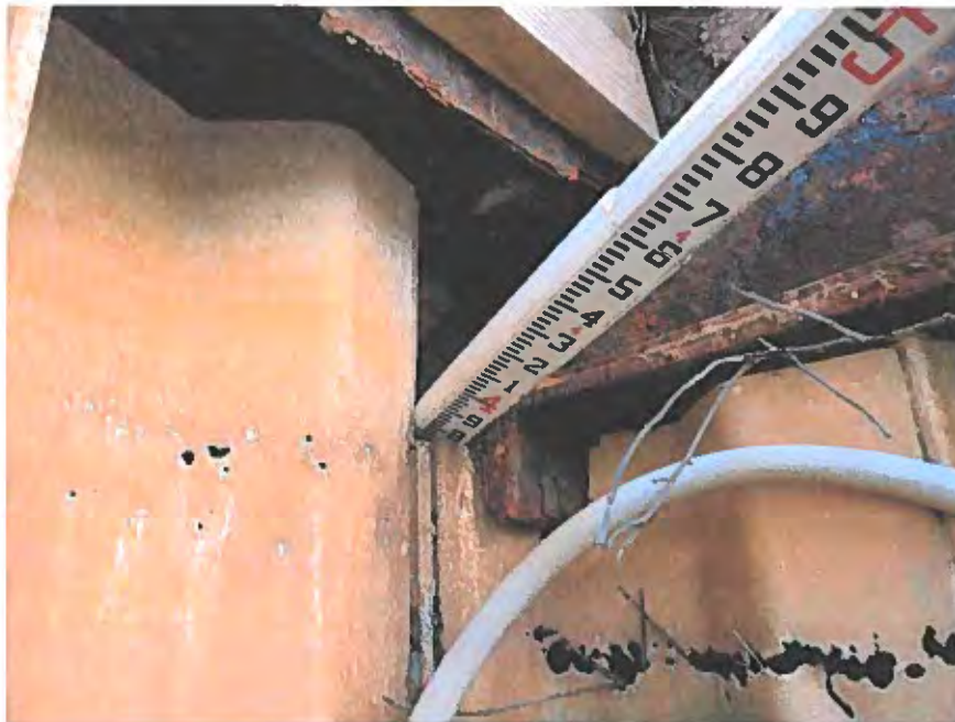
PHOTO 10 –SLAB UNDERMINING – UP TO 4 FT NORTH SIDE
