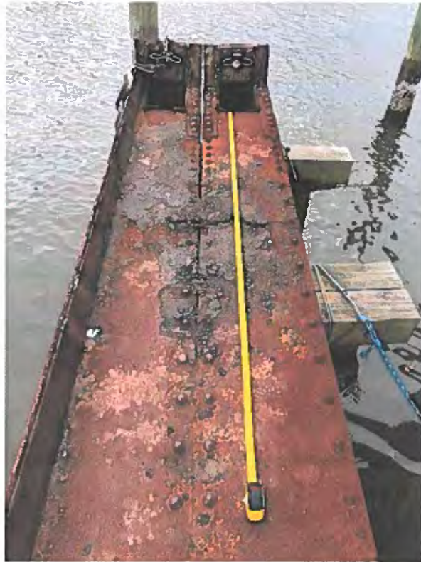
PHOTO 1 -FINGER PIER NO. 1 –BEAMS A AND B SECTION LOSS IN TOP PLATE
