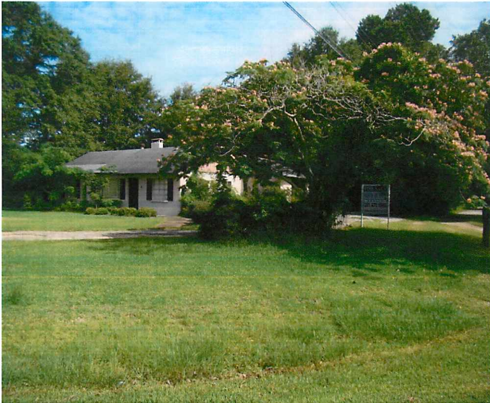
View of Subject Property from Greeno Road.
