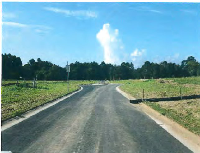
View to the South on Hemlock Drive
