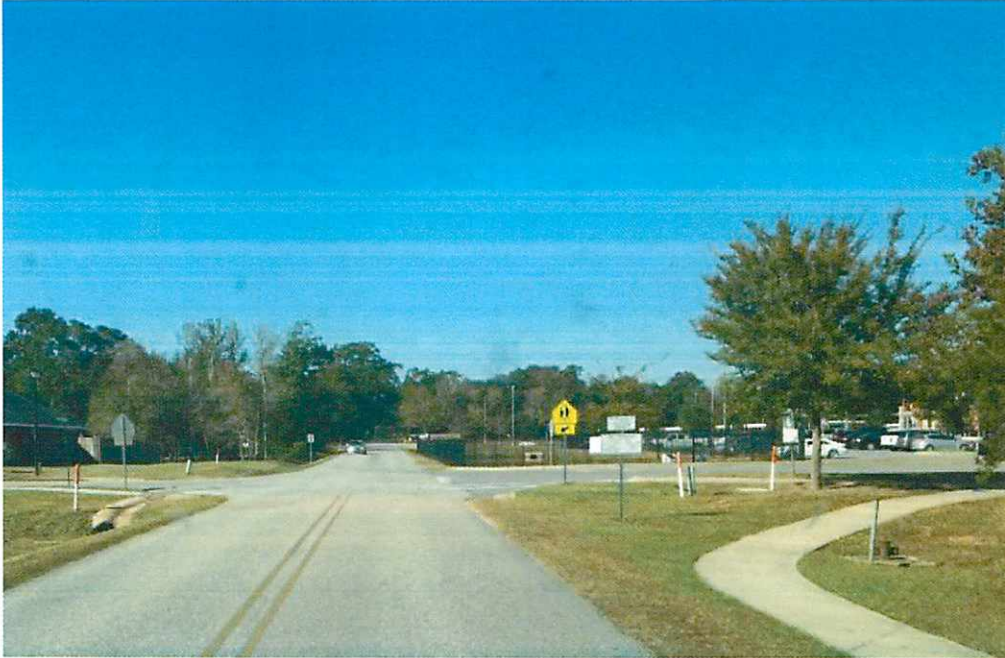
PICTURE 5 – MANLY RD LOOKING WEST TOWARDS HWY 98 APPROACHING THE FIRST DRIVEWAY TO FAIRHOPE MIDDLE SCHOOL
