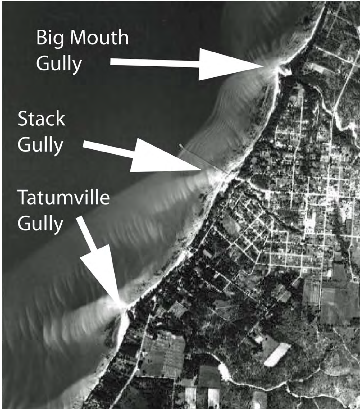
Figure 2: Aerial imagery of Fairhope's beaches (1938) showing major gullies entering Mobile Bay.
