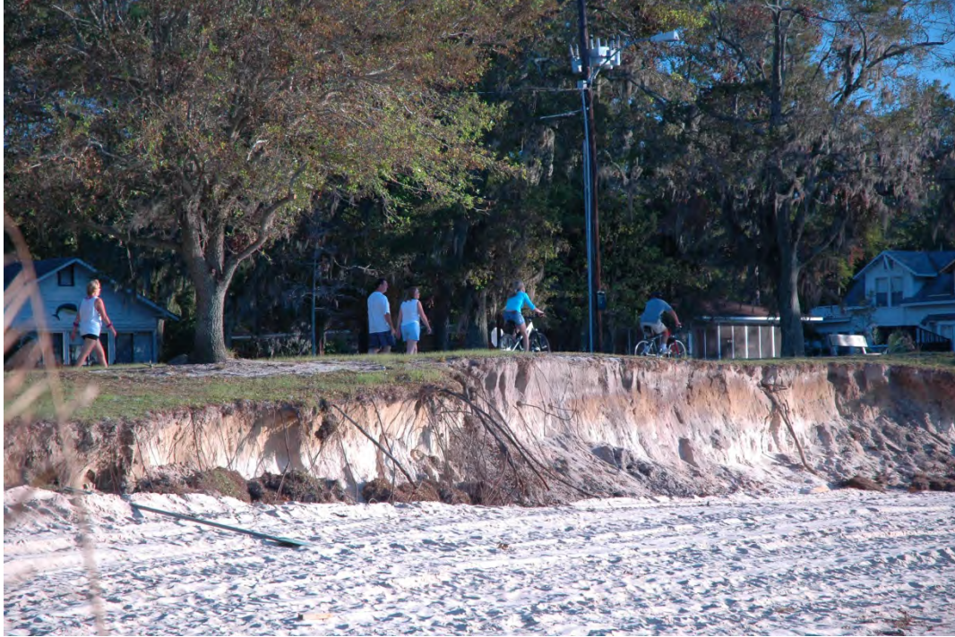
Figure 5: October 2004 photograph shows that some sand (unknown quantity) was mechanically placed on the beaches in the foreground at the northern end of Magnolia Beach Park after bluff erosion exacerbated by Hurricane Ivan (Also: note the small live oak tree on the bluff in the background on the left side of the photograph. That tree was destroyed a year later by bluff erosion caused by Hurricane Katrina)
