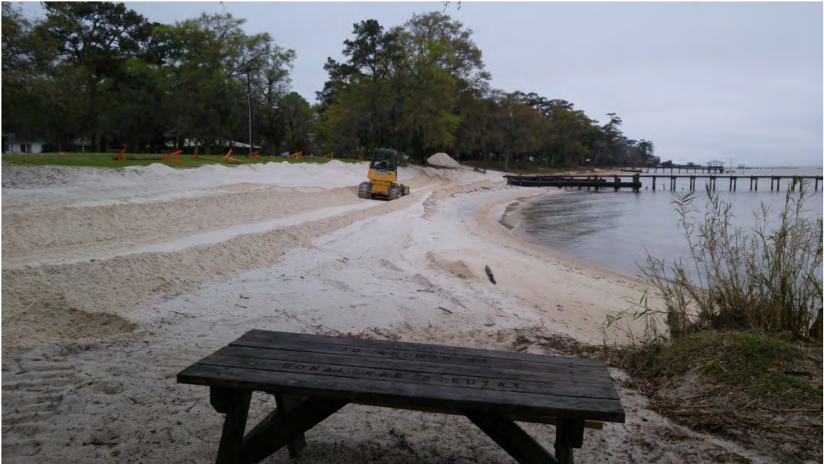
Figure 6: Photograph showing new sand being spread at Magnolia Beach Park in the 2016 beach nourishment (March 2016).
