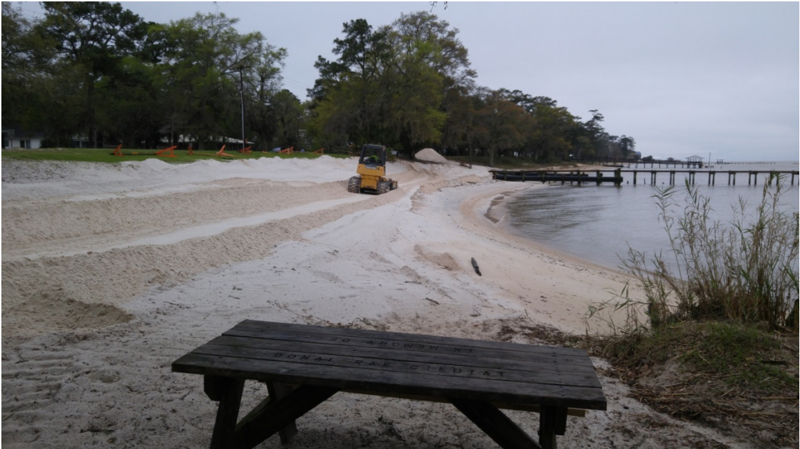
Figure 6: Photograph showing new sand being spread at Magnolia Beach Park in the 2016 beach nourishment (March 2016).
