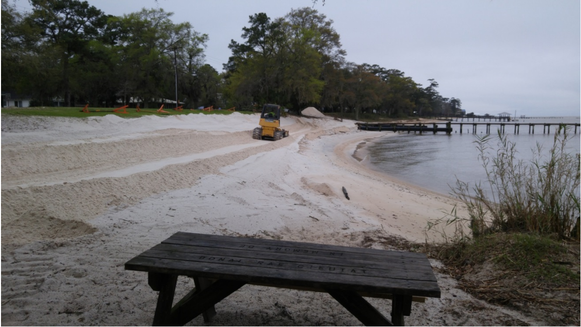
Figure 6: Photograph showing new sand being spread at Magnolia Beach Park in the 2016 beach nourishment (March 2016).
