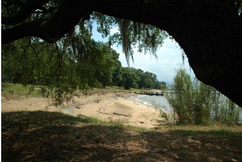
Figure 3: Photograph from June 2004 showing that bluff erosion at the north end of Magnolia Beach Park was problematic in early 2004. This photograph was taken looking south through the overhanging limbs of the large live oak tree which is south of the boat ramp. (Note: In 2004, the roots of that tree in the center of this photograph were exposed by the erosion – see Figure 4).
