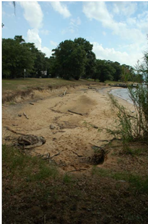
Figure 4: Photograph from June 2004 showing exposed roots of the large live oak tree near the boat ramp. This beloved oak tree still exists today because of the beach nourishments and the timber headland-jetty structure constructed in 2005 to its immediate southwest
