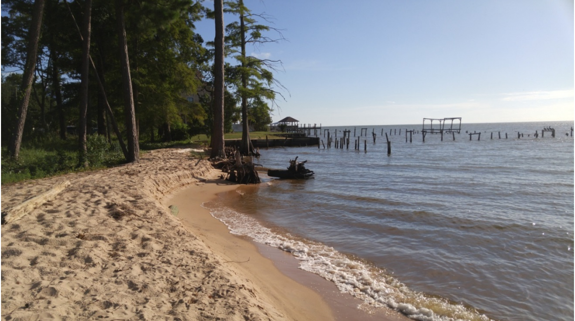
Figure 14: Photograph (facing south) showing summer erosion at the southern end of Magnolia Beach Park, near the American Legion (July 2016).
