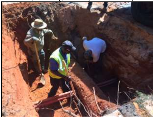
Pictured: Storm drain pipe replacement on Fairhope Avenue
