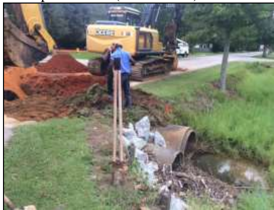
Pictured: Fairhope Avenue pipe extension (near CR 13)
