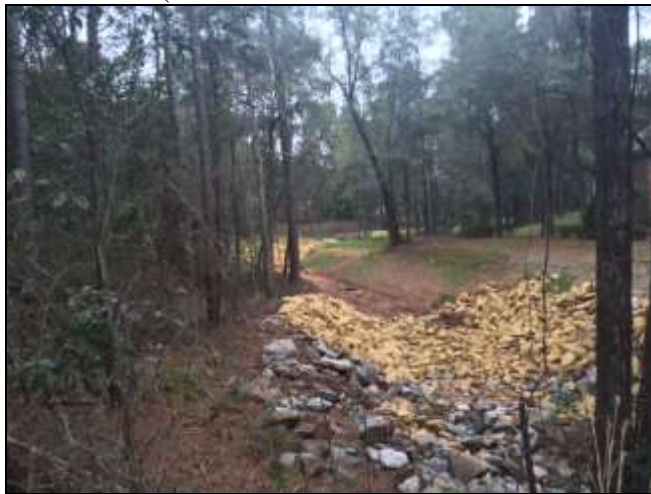
Pictured: Woodlands Drainage Project
