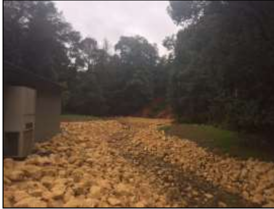
Pictured: Treatment Plant Stream Bank Stabilization
