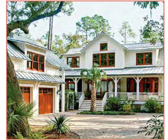
Garages should not dominate the streetscape. Front-loaded garages should be located to the rear, side-loaded, or recessed from the front facade
